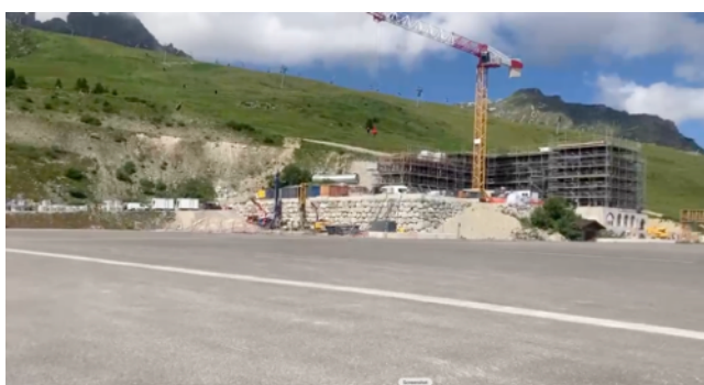
Construction tower crane on the airfield.
