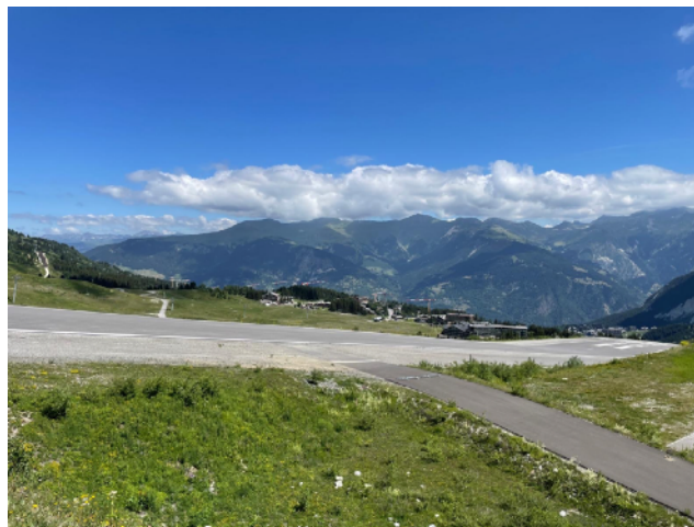
The 18.5% runway slope of Courchevel.
